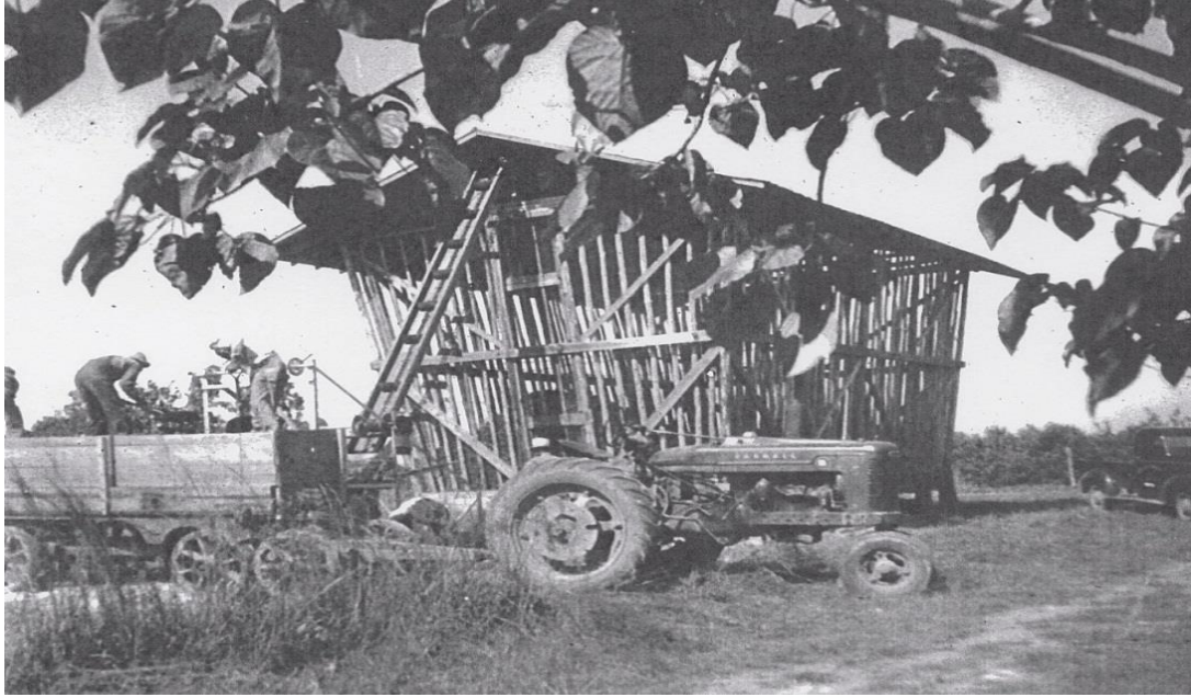
Figure A.11 Tung nut drying shed
